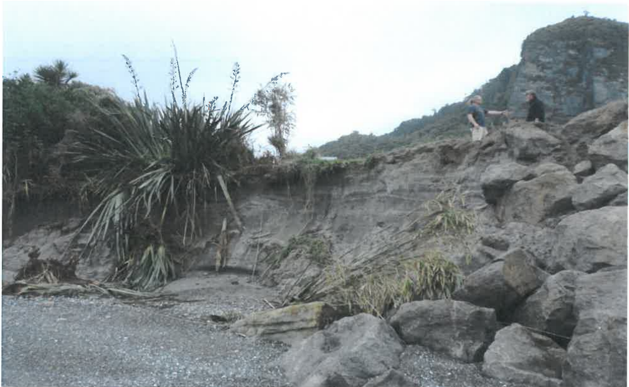
Erosion bite at northern end of wall. 15 March 2016.
